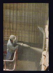
Pre-blended dry or damp materials are placed into the delivery equipment. Compressed air conveys material through a hose at high velocity to the nozzle, where water is added. Material is consolidated on the receiving surface by the high-impact velocity.
