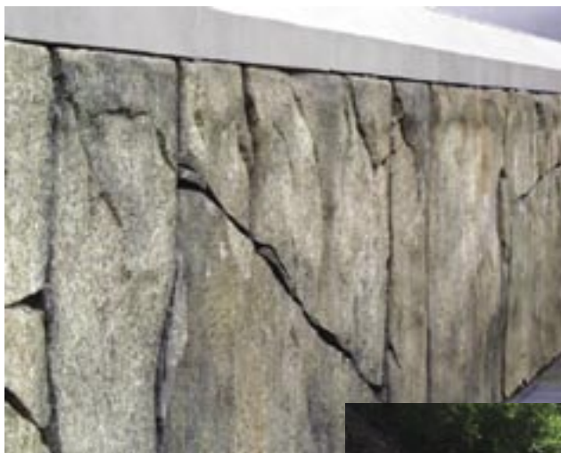
Fig. 1: Granite rock finish at retaining walls of a home built on Lake Washington, Seattle, WA. This type of finish is a good alternate to a stone veneer
