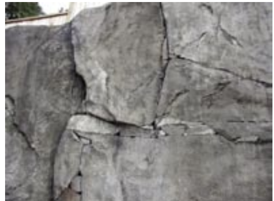
Fig. 8: Close-up of carved granite. SE 228th Street retaining wall, Sammish, WA, was the Washington Aggregate and Concrete Association Artistic Merit award winner
